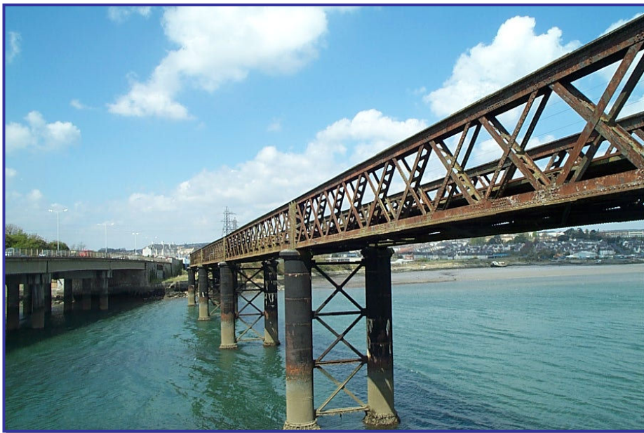
Figure 1 Laira Rail Bridge
